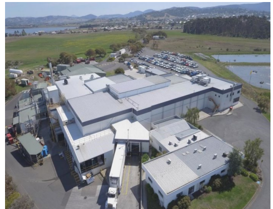
Poultry Processing Plant.
